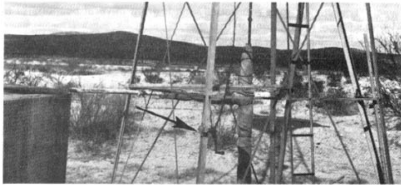
Windmill. Note windlass (arrow).
