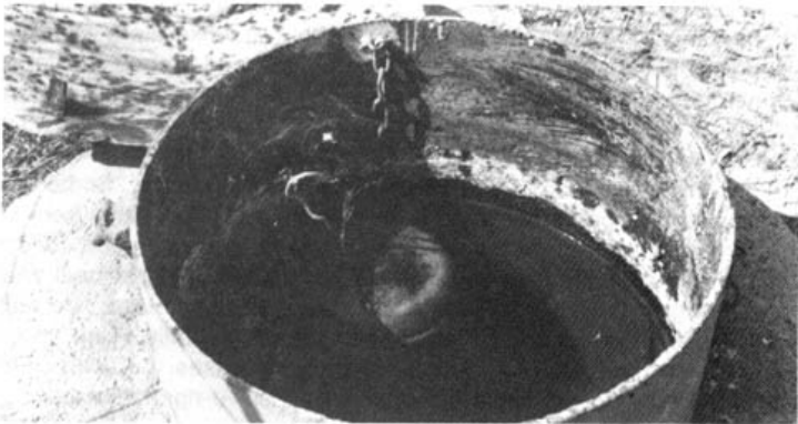
Float-valve regulates water level in stock tank.
