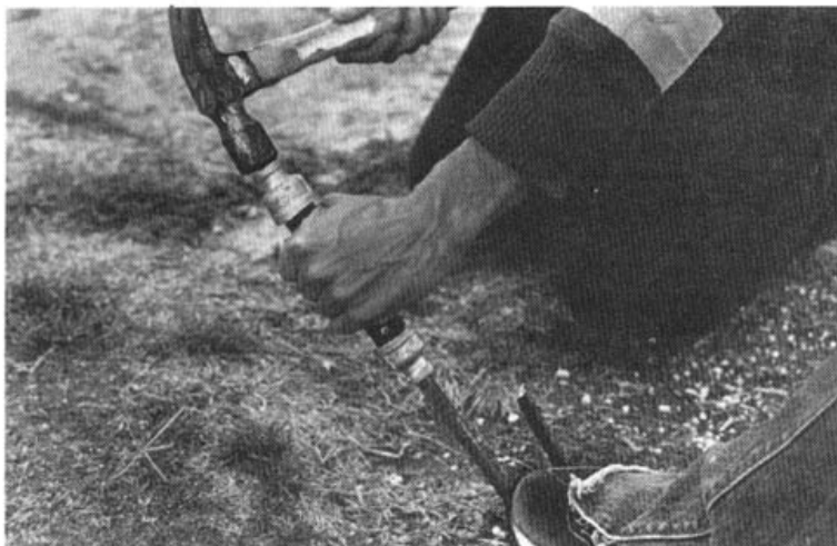
Place the driver over the sharpened end of the rebar stake and hammer it in.
