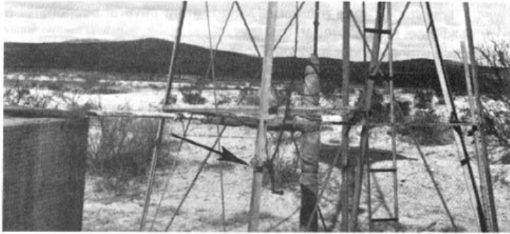
Windmill. Note windlass (arrow).
